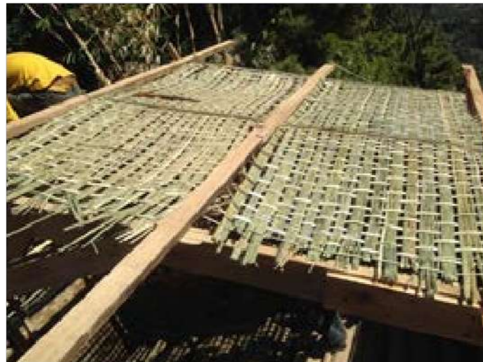
Local material 'Mandro' below CGI roofing for thermal insulation
