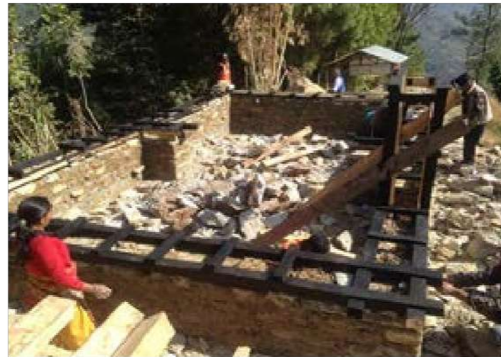
Wooden seismic band installation
